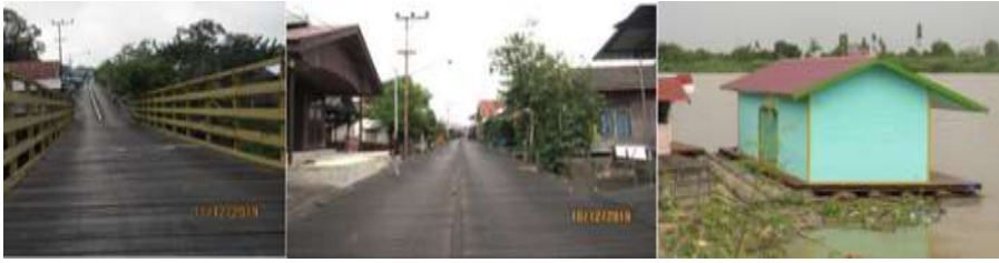
Fig. 4. Ironwood used for village infrastructure. Left to Right: Bridge, Boardwalk and Pontoon for boat house. Source: Doc. Nurjanti, 2019
