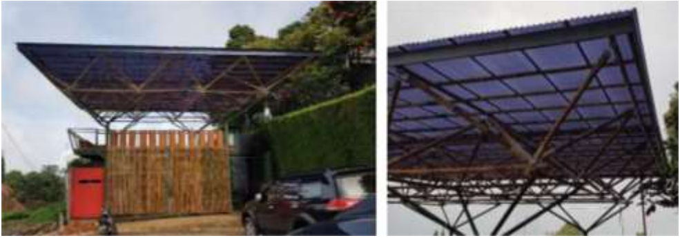
Figure 2. Implementation of Bamboo Space Frame
